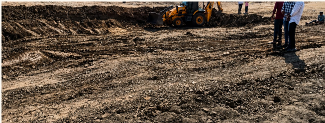
Desilting a village pond, April 2026. The silt goes onto the fields; the deepened pond takes the next monsoon. Eleven sites were done this way.
