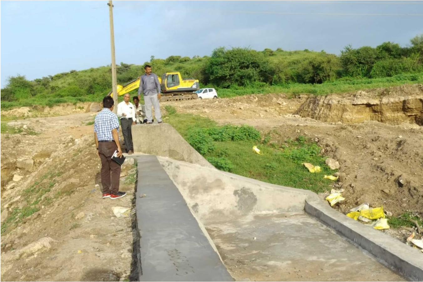
Mota Umarda check dam, August 2025 – the spillway concreted, the excavator still on site. Twenty-six structures like this were renovated across the year.
